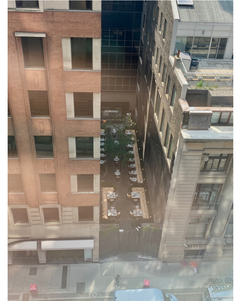
Aerial view of Daphne Restaurant Patio from our office on the 9th floor at 80 Richmond St W
