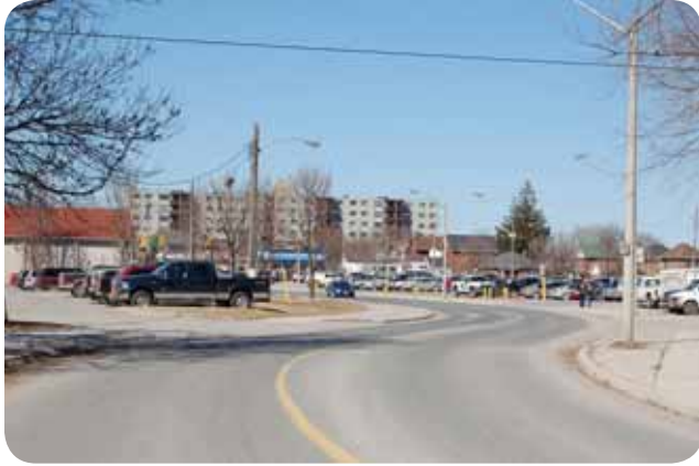
Roger Neilson Way looking north
