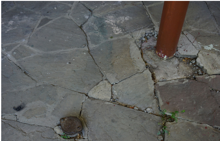
FIGURE B-27 Flagstone pavement detail at column support
